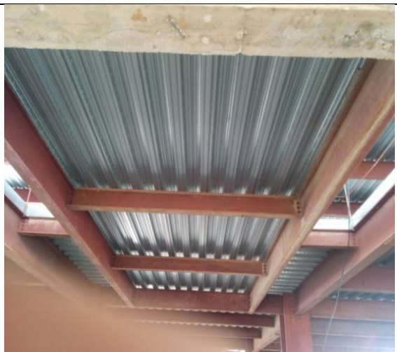
FIGURE 1.5 (e) Bottom view of Decking
