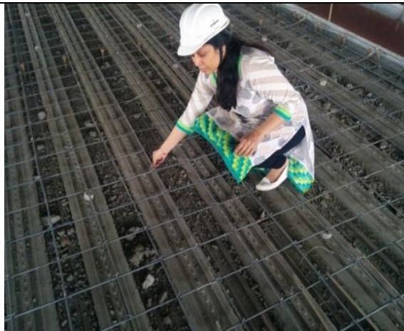
FIGURE 1.5 (c) Secondary Bars
