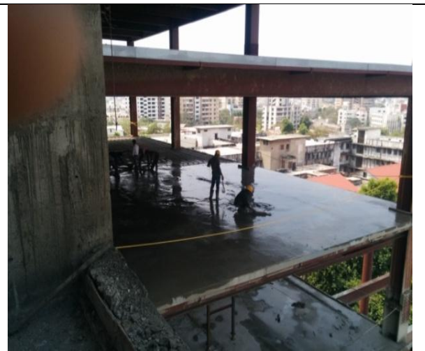
FIGURE 1.5 (f) Finishing of Concrete
