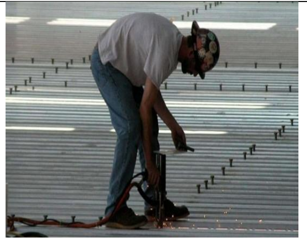
FIGURE 1.5 (b) Installation of Studs [54]
