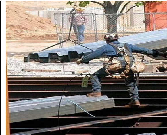
FIGURE 1.5 (a) Decking Installation [54]
